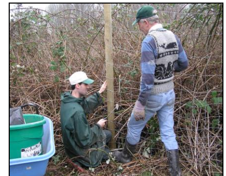
Installing further deer fencing
